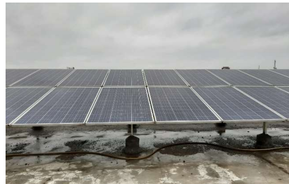
10KWp ROOFTOP SOLAR PV PANELS
