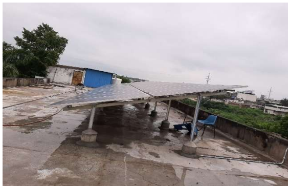
10KWp ROOFTOP SOLAR PV PANELS
