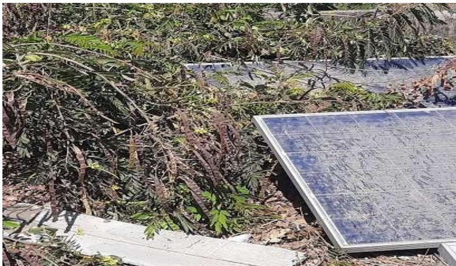
Fig: UN-UTILISED SOLAR PANELS PORTION (COVERED BY TREE)
